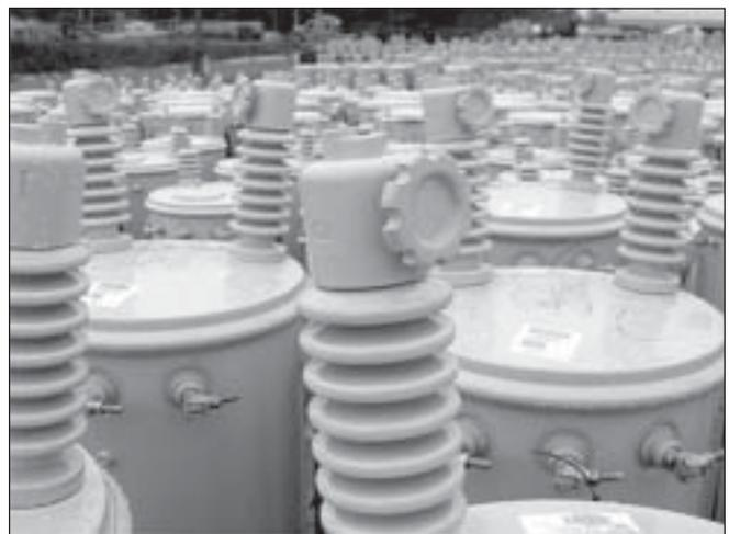
Figure 2: 2140 Wildlife Protectors installed on overhead distribution transformers.
