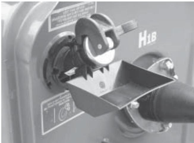
Figure 2: Drip Guard installed in a single-phase pad-mounted transformer.
